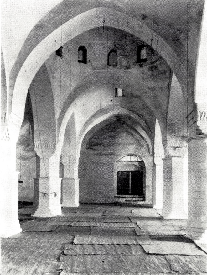
Ḥama, Great Mosque. Interior of prayer hall as seen towards the west. — In back wall the central door of the Byzantine church and above left at abutment of vault an irregular projection. — Phot. B. HORNEMANN 1933.
